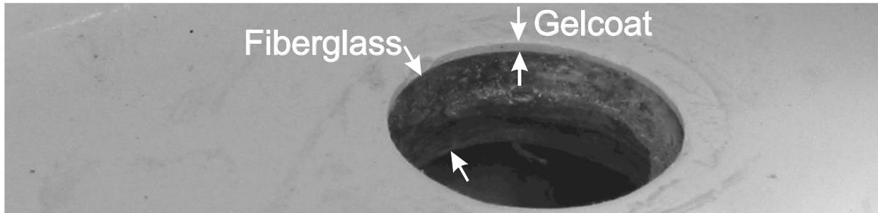
The gelcoat is a very thin layer approximately 1/16<sup>th</sup> thick and the fiberglass below it is normally about 3/8" thick. IMPORTANT: If the fiberglass below the gelcoat is less than 3/8" thick, you need to add fiberglass cloth and/or marine treated plywood to build up the largest area available to at least 3/8" thick. You need to check all mounting points as the fiberglass thickness may vary on the boat.
